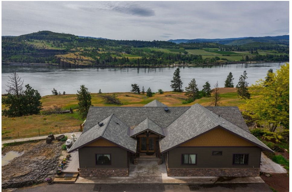
FIGURE 1: CATHERINE CREEK RESIDENCE
