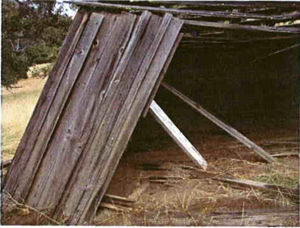
Photograph 23: Left side of South elevation
