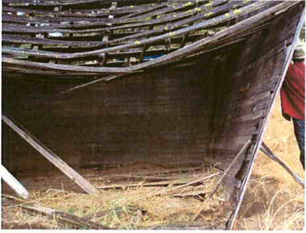
Photograph 24: Right side of South elevation
