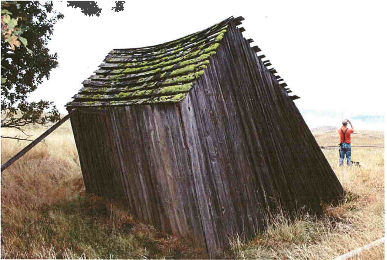
Photograph 4: View to the Southeast
